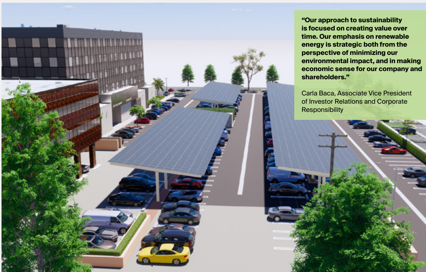
Solar Carport Project, West Hills, CA
