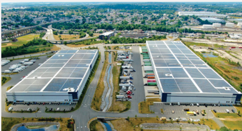
Perth Amboy, New Jersey Community Solar Panels
