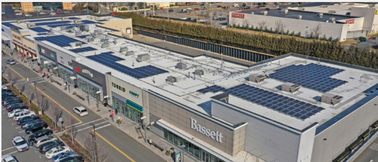
Chimney Rock Solar Panels
